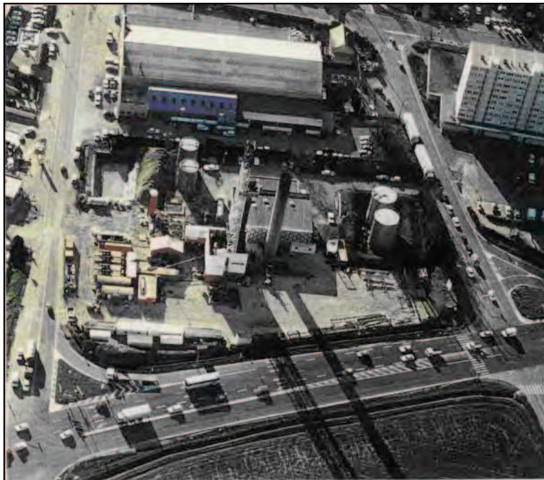
Fig.10.5. Aerial view of a drilling site in the Paris suburban area (GPC and Sedco-Forex, 1995)
